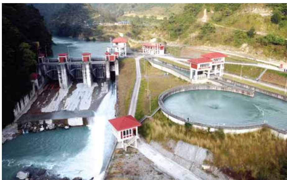
The Upper Marsyangdi-A Hydropower Project in Bhulbhule, Lamjung, highlights the long-term challenge of building infrastructure to withstand an increasingly unpredictable Himalayan environment. Photo: Global Carbon Council (GCC)
