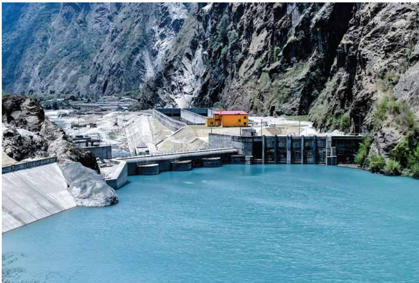
The Upper Tamakoshi Hydropower Project in Dolakha, Nepal, reflects the Himalayan region's vast hydropower potential and the risks of building infrastructure in its rugged terrain. Photo: Upper Tamakoshi Hydropower Project
