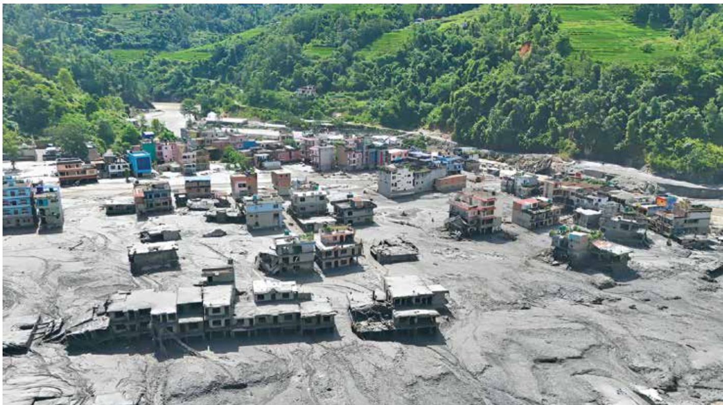
The Rasuwa disaster exposed the vulnerability of hydropower infrastructure to extreme mountain hazards. Photo: Hemanta Shrestha/TKP
