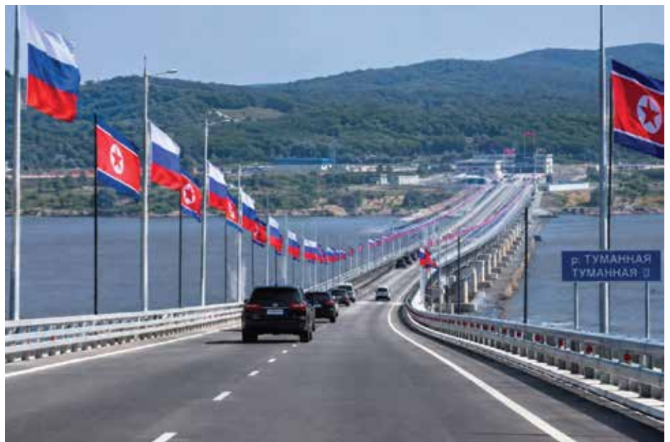
A new road bridge links North Korea's Rason region with Russia's Khasan, reflecting the countries' expanding economic and logistical ties. Photo: Armenpress
