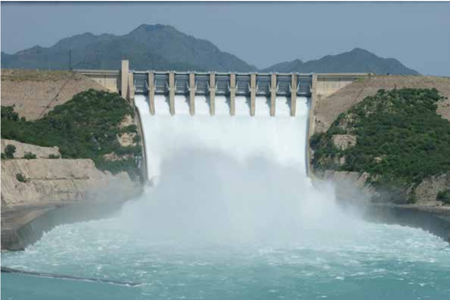
Tarbela Dam on the Indus River is a major part of Pakistan's water infrastructure, supporting irrigation and water security downstream.
