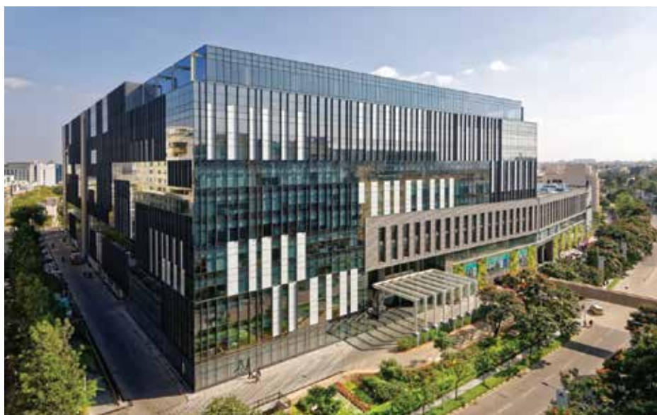
Manyata Tech Park in Bengaluru, one of India's largest technology hubs, reflects the country's efforts to adapt its IT sector to the AI era. Photo: MFAR
