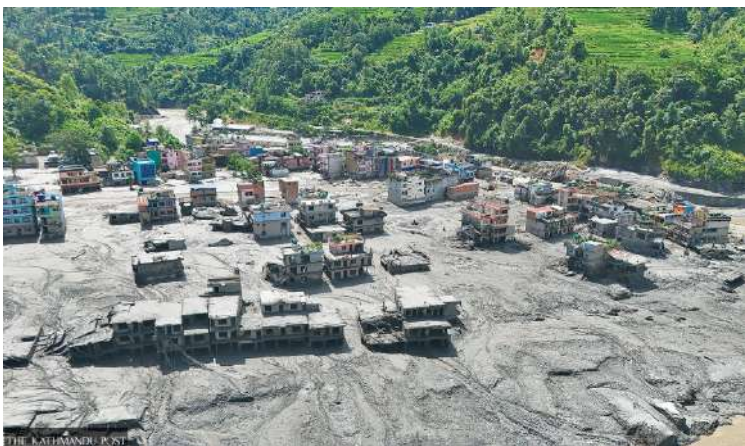
The Rasuwa disaster exposed the vulnerability of hydropower infrastructure to extreme mountain hazards. Photo: Hemanta Shrestha/TKP
