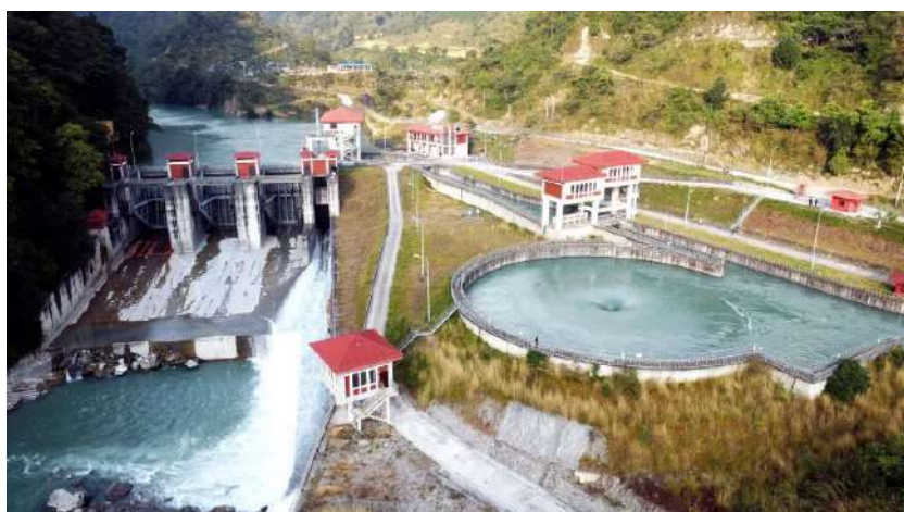
The Upper Marsyangdi-A Hydropower Project in Bhulbhule, Lamjung, highlights the long-term challenge of building infrastructure to withstand an increasingly unpredictable Himalayan environment. Photo: Global Carbon Council (GCC)
