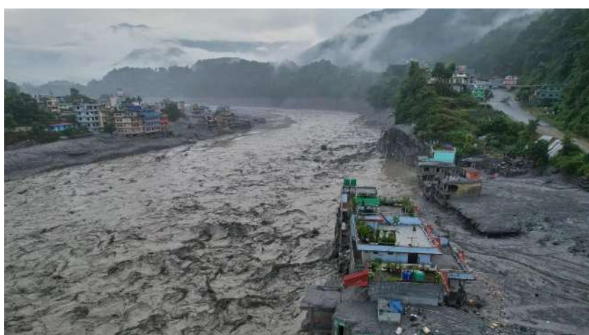
A drone view of the aftermath of flash flooding along the Trishuli River in Nuwakot, Nepal, highlighting the extreme hazards facing infrastructure in the Himalayan region. Photo: Rajesh Kumar Singh/AP Photo
