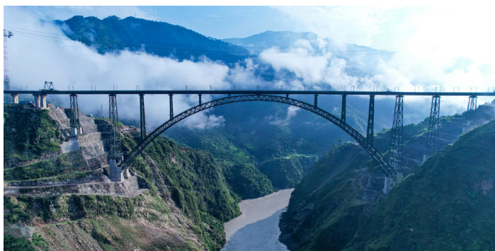
The Chenab Bridge spans the Chenab River in Jammu and Kashmir, one of the western rivers at the centre of India's water-sharing dispute. Photo: COWI
